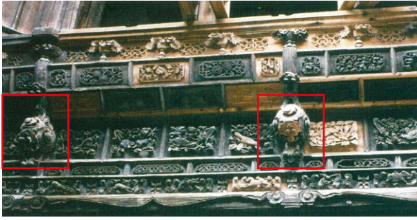
fig. 4 Detail of a balcony located in the Chengshi Sanzhai [The Three Mansions of the Cheng's], Huangshan city, Anhui province 圖四 安徽黃山程氏三宅陽台外牆如意捲葉足雕刻細圖
